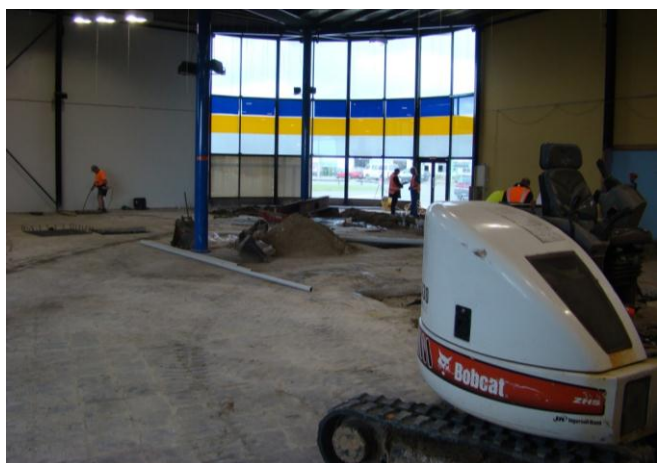
Concrete is being dug up and key services are being installed
